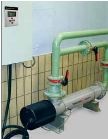
The highly efficient "L-shaped" design and LPHO amalgam lamps result in an extremely compact footprint.
