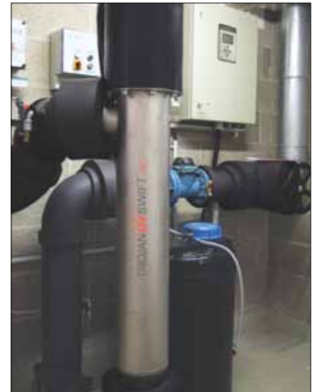
The highly efficient "L-shaped" design and LPHO amalgam lamps result in an extremely compact footprint.
