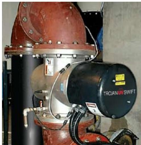
*Developed in consultation with Operators and Consulting Engineers, the TrojanUVSwift™ is extremely space efficient. Its compact footprint allows the system to be integrated into restrictive pipe galleries of water treatment facilities – reducing installation costs and eliminating the need for larger buildings or additions.*
