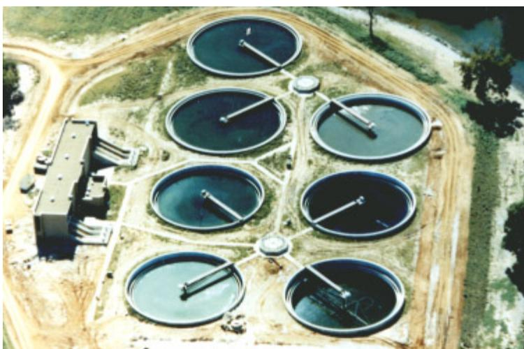
*The four, 110 ft. Kraus Fall Clarifiers (seen in the foreground) provided BOD<sub>5</sub> removal in stage one. The three, 122 ft. stage two clarifiers (seen at back) provided nitrification for an average design flow of 20MGD through each stage.*
