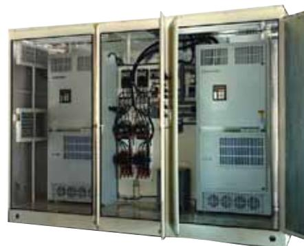
*VFD duplex 200 hp pump control package with air conditioning*
