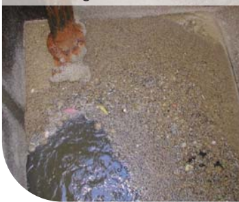
Ft. Collins, Colorado After: < 1" grease
