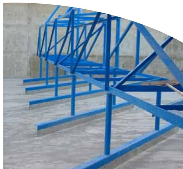
The C3D is equipped with a scum skimmer system. Ovivo offers a standard scum box with skimmer blades supported by rake arms or an enhancing skimming design with a full trough skimmer (FTS) and two cantilevered skimming blades.
