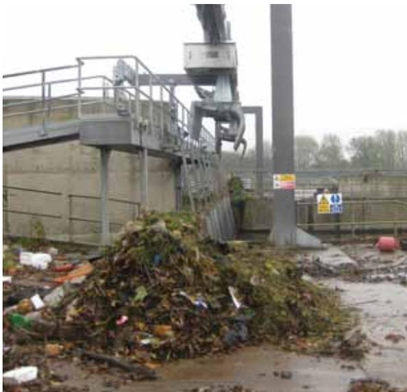
Ovivo designed, manufactured and installed the above Brackett Bosker® Overhead Trashrake with two machines on a common track each with a 3,000kg lifting capacity
