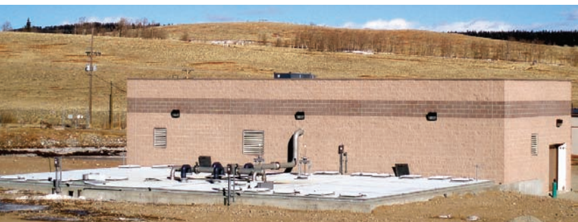
The covered clarifier basins behind the treatment plant.
