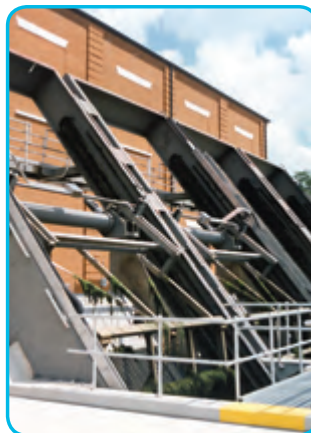
STORM DRAINAGE PUMP STATION
