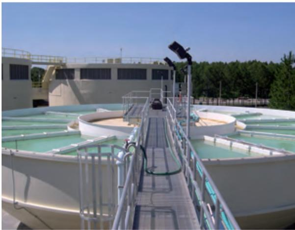
A recognized leader in its class, Infilco Degremont's Accelator® Clarifier is a high-rate treatment plant in a single basin that employs the principle of internal slurry recirculation.
