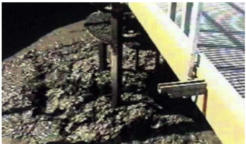
Draft Tube Installation - Mixing 4% Solids
