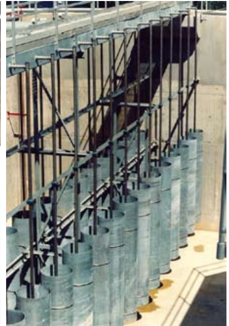
Shear Tube Installation - 24-ft. Deep Basin
