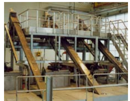
Integrated DSP for de-watering effluent
