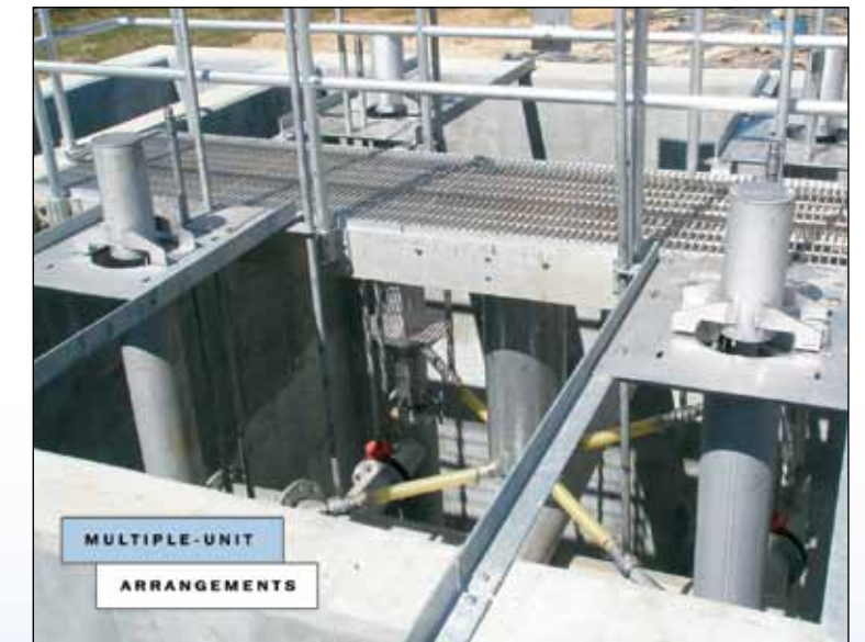
Multiple-unit Strata-Sand™ sandfilters are available for high-throughput applications. Usually four or more filter modules are built in one concrete filter basin, to suit the required flowrate.
