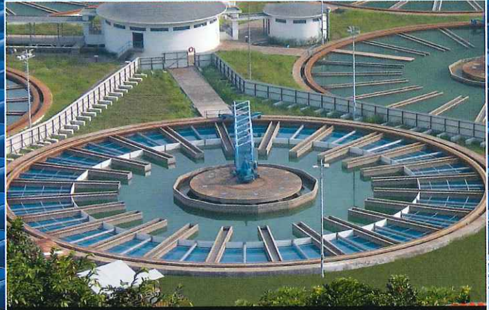
Sha Tin Water Treatment Works, Hong Kong, China
